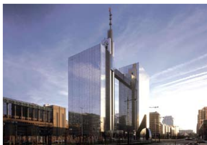
Belgacom Towers – arch. M. & J-M. Jaspers - J. Evers & Partners
